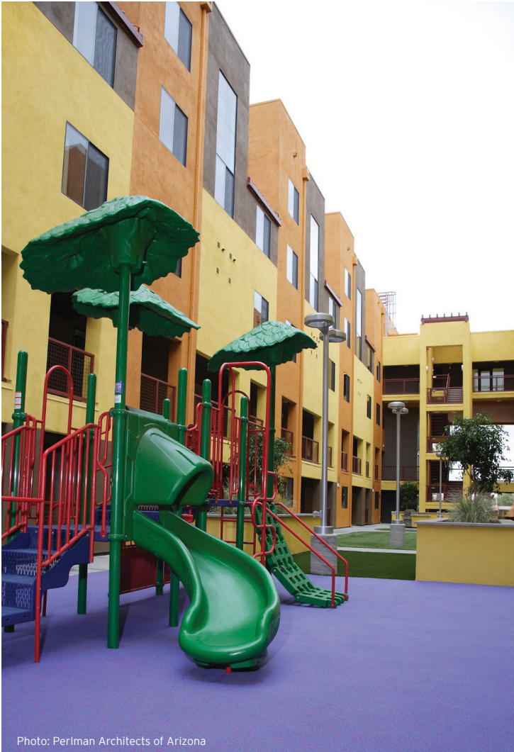
Photo: Perlman Architects of Arizona
