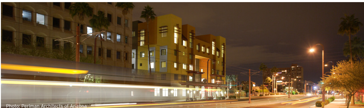
Photo: Perlman Architects of Arizona
